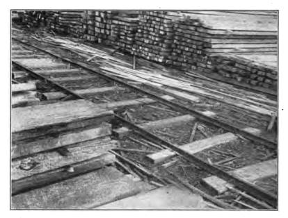
Fig. 87.—Piling sticks lying on the ground at a mill in South Carolina, showing the insanitary method of handling them. Such sticks lying for only a week or two in contact with fungus-infected ground may themselves become seriously infected, and may in turn pass the decay on to the lumber stacks.
